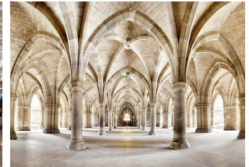
Glasgow University Cloisters
