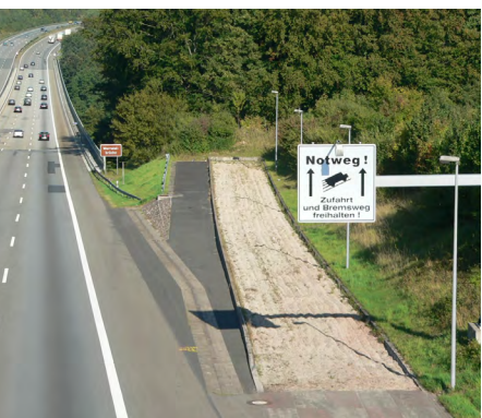
Truck arrester bed on highway in South Korea (top) and Germany (bottom)
